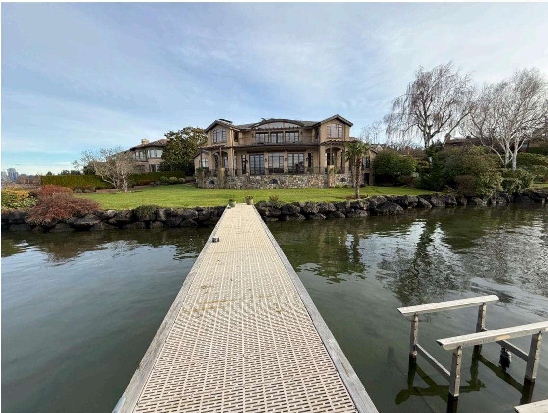
Photo 2 - Existing dock looking shoreward showing bulkhead to be replaced.
