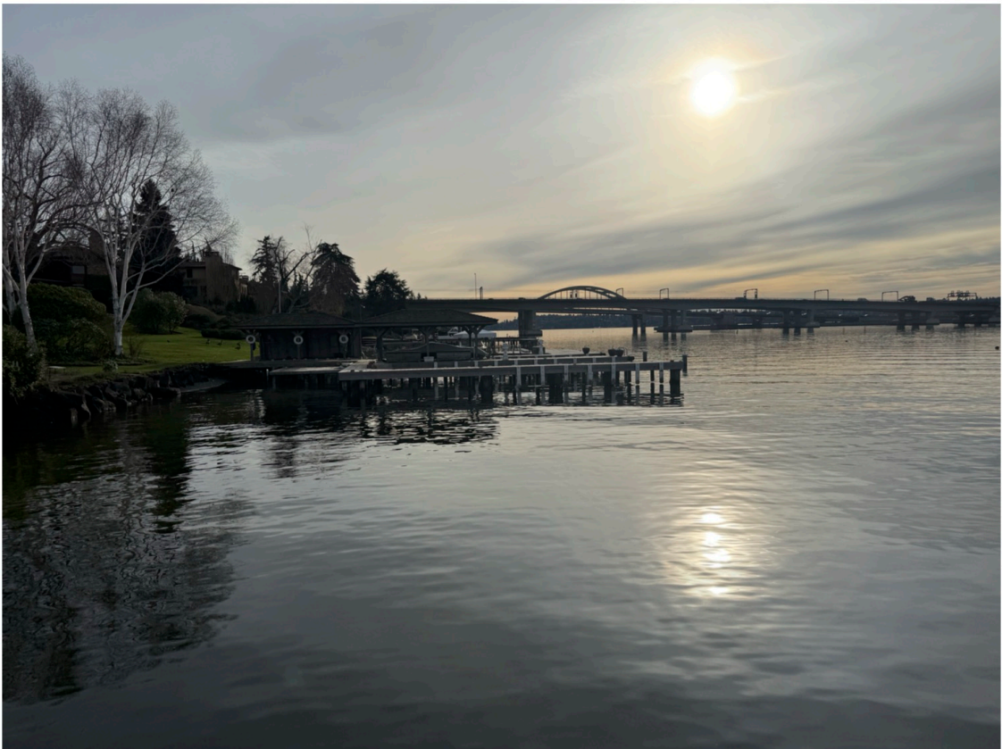
Photo 6 - Conditions south of the site.
