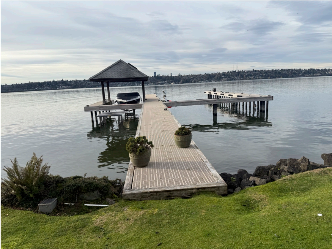
Photo 1 - Existing dock looking waterward.
